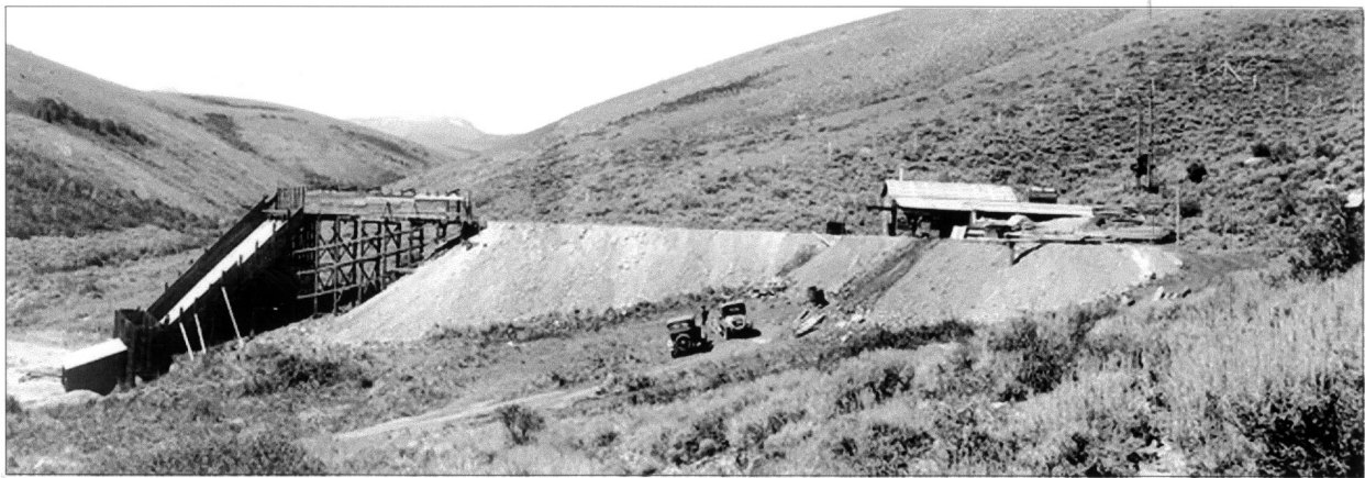
Figure 39. Bear Lake Mine, August 30, 1920. Photo by G. R. Mansfield, #476, 477, USGS Photographic Library.
